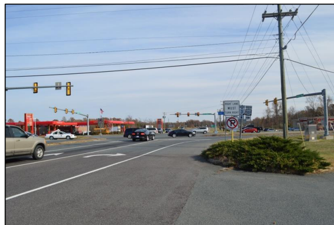
ROUTE 3/301 INTERSECTION IN KING GEORGE COUNTY
