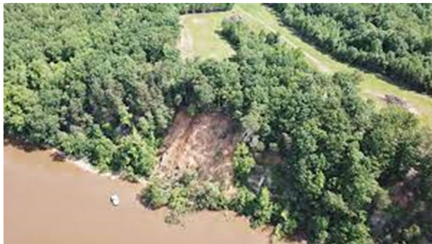
Figure 6-12: Fones Cliffs Landslide May 24, 2018
